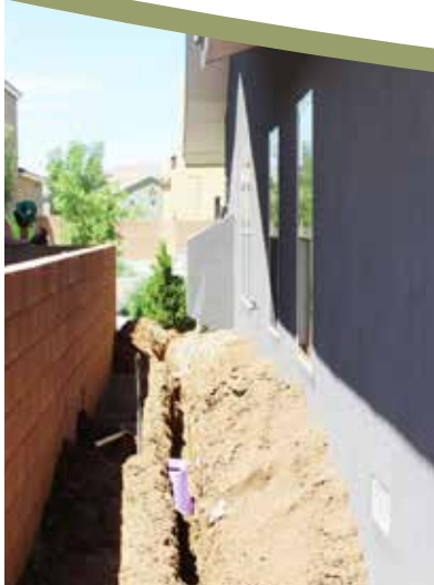
2. TRENCHING TO CONNECT IRRIGATION
