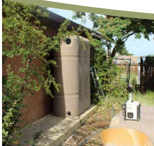
2. LEVEL PLATFORM FOR TANKS
