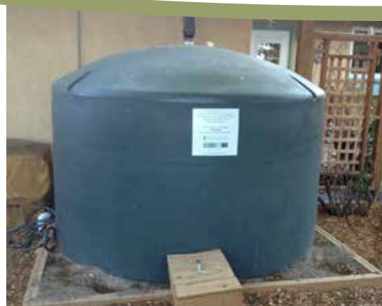
3. INSTALLED 1650 GALLON CISTERN TANK
