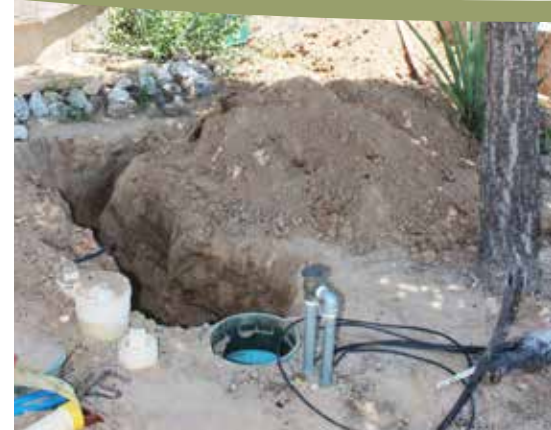
3. INSTALLING PIPING TO TANKS
