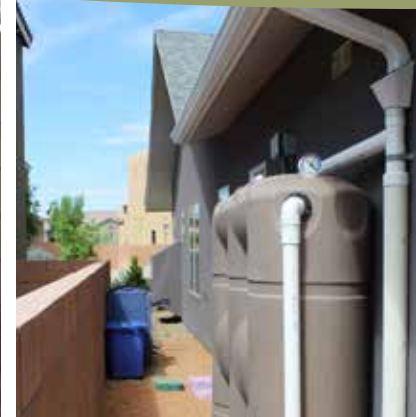
4. INSTALLED 530 GALLON CISTERN
