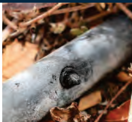
GOOF PLUG REPAIR ON POLY LINE
